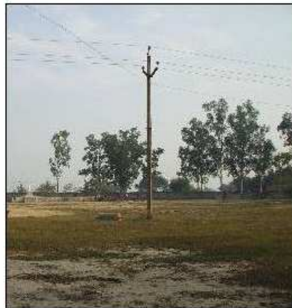
10 EXISTING ELECTRICAL LINE & POLE TO BE RELOCATED
