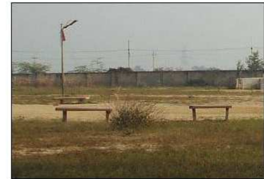
11 EXISTING STREET LIGHTS TO BE REMOVED
