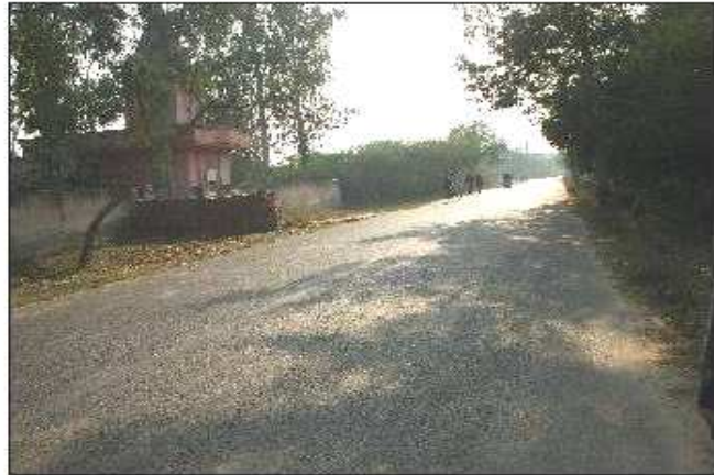
① 15 MTR WIDE MAIN APPROACH ROAD FROM THE NAGAFGARH VILLAGE SIDE
