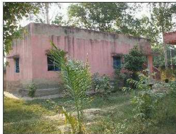
④ EXISTING HALL TO BE DEMOLISHED
